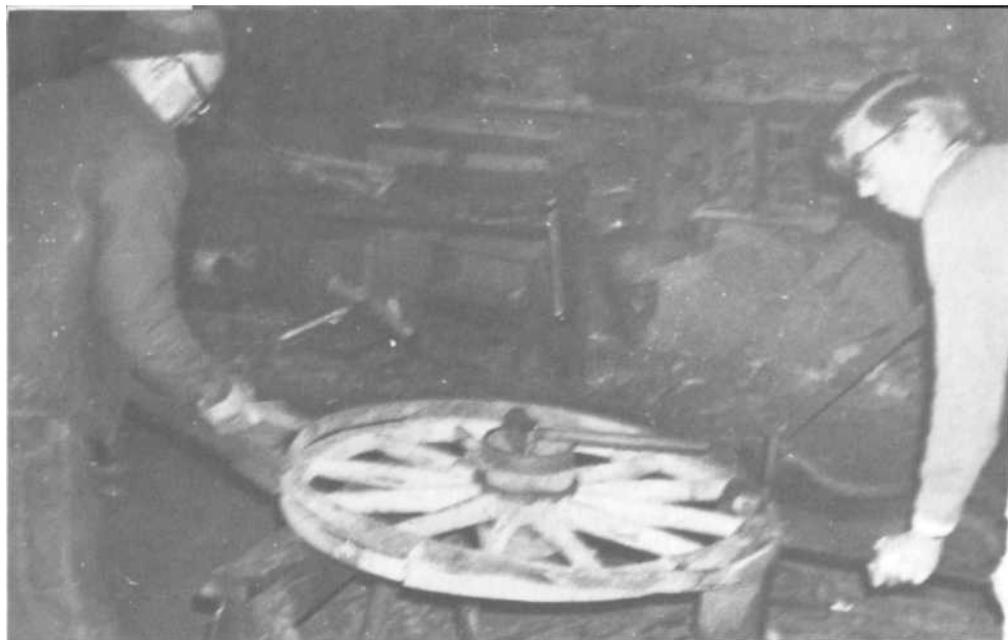
PLATES 111—113 Moving quickly, he carries the tire to the wheel, has a second person clamp down on the opposite side to keep the tire from flipping up (Plate 111), and pulls the tire over the rim of the wheel with a "tire puller" (Plates 112-113).
