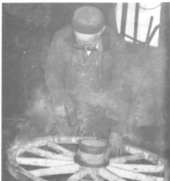
PLATE 114 As the wood smokes from the heat, he pounds the tire down evenly all the way around and douses it repeatedly with water to finish the job.
