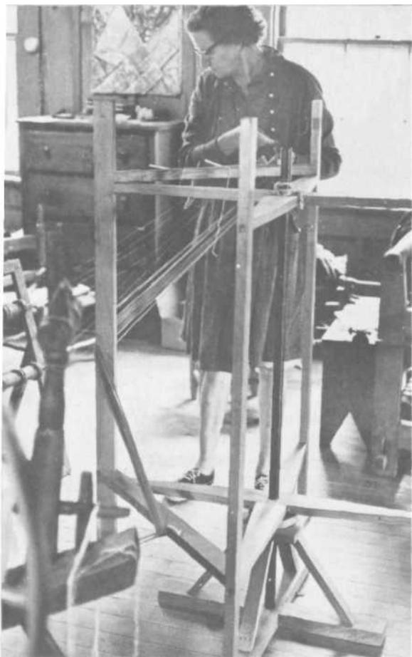
PLATE 249 Dean uses a WARPERS like the one shown here rather than use the more traditional warper described later. One revolution of the warper (bottom peg to top peg) equals three yards. When Dean weaves a three-yard piece the width of a stole (230 threads), she mounts ten spools in the spool rack, and goes from top pegs to bottom pegs twenty-three times. As each spool runs out, she mounts a full spool in its place, ties the thread ends together, and continues.
