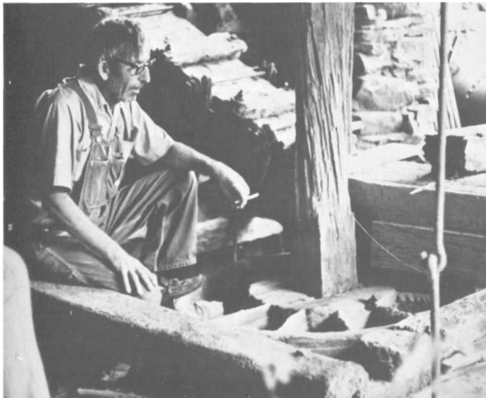
PLATE 160 Sharpening millstones as they get worn through use is one of the trickiest jobs involved in running a mill. The fans are recut periodically by slowly and painstakingly pecking away at them with a hammer like the one Sam is using. Sam never "beats" on the rock—he just taps lightly hour after hour until the sloped surfaces of the fans are just right.
