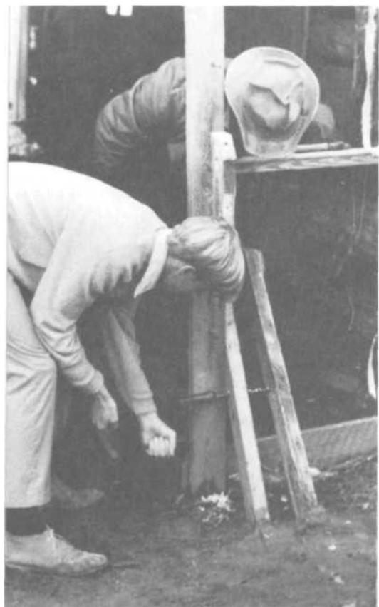
PLATE 172 The pedal itself is a two-foot-long 2X4, a hole drilled through it six inches from one end. It is set in place between the two braces, and held by a bolt that goes through it and the two holes Greg drilled in the braces. With the pedal in place, one end of the deerskin rope is wired to the center of the pedal.
