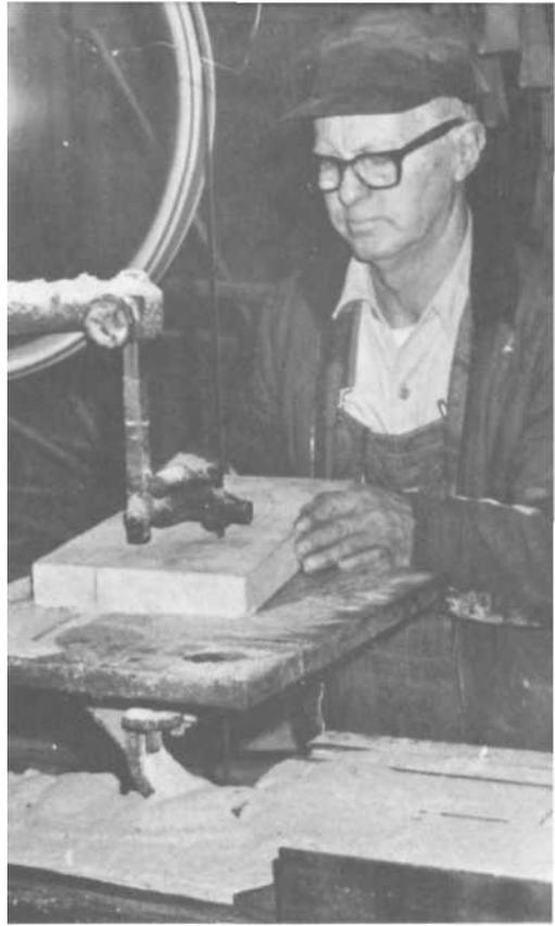
PLATE 95 He drills the holes for the ends of the spokes with a drill press, rather than with the auger which would have been used traditionally. He drills the holes from the inside of the felloe.
